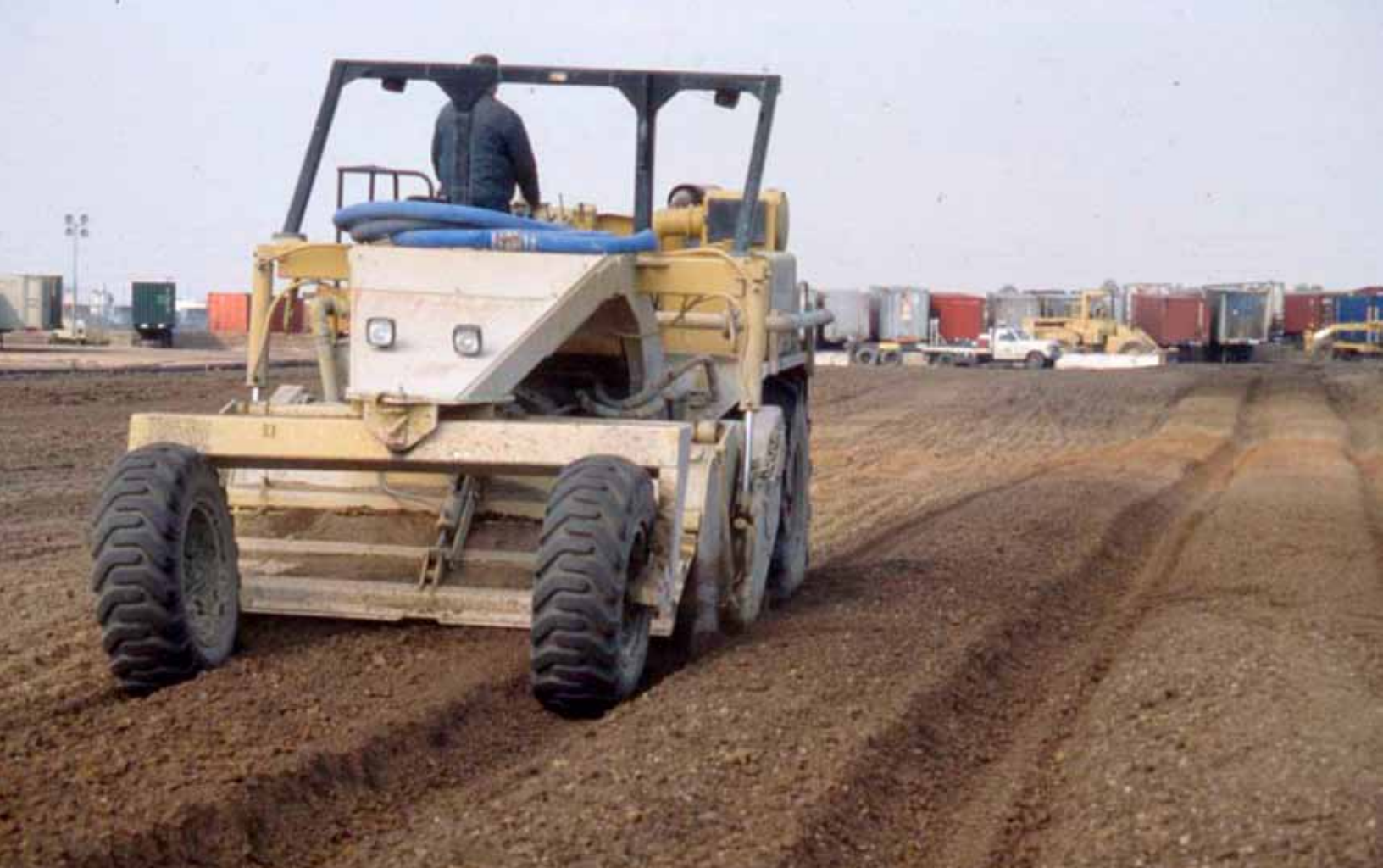
EMC SQUARED BEING MIXED WITH NATIVE SOIL ▲
