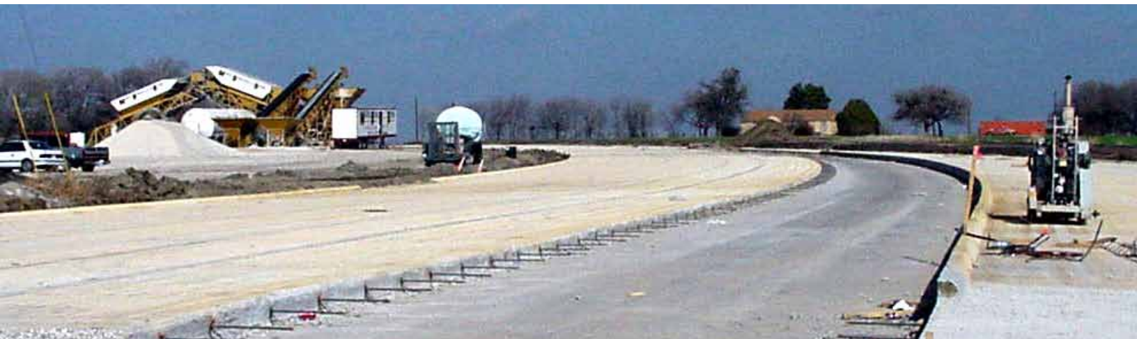
Concrete Batch Plant with Concrete Placement in Progress
