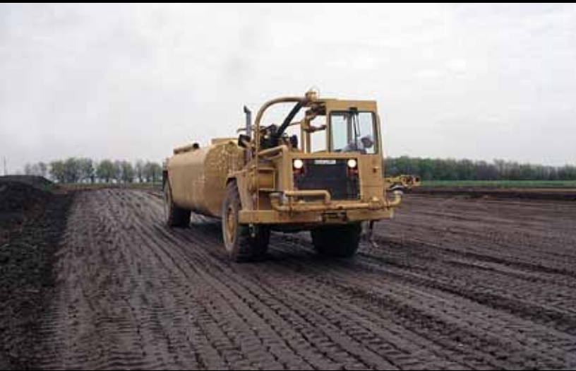
Rubber Tire Rolling of Working Platform Surface
