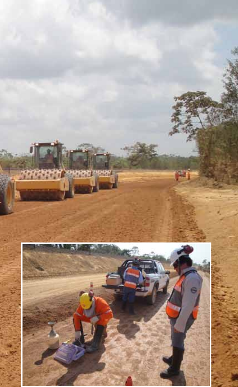
Compaction Testing of EMC SQUARED System Stabilized Subballast Layer
