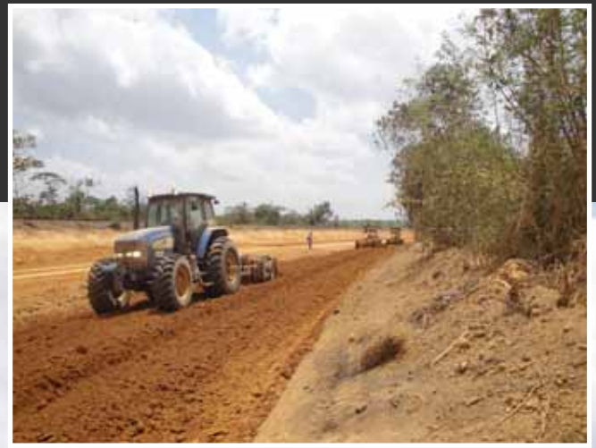
Mixing of EMC SQUARED System Stabilizer Solution with Subballast Soil Materials
