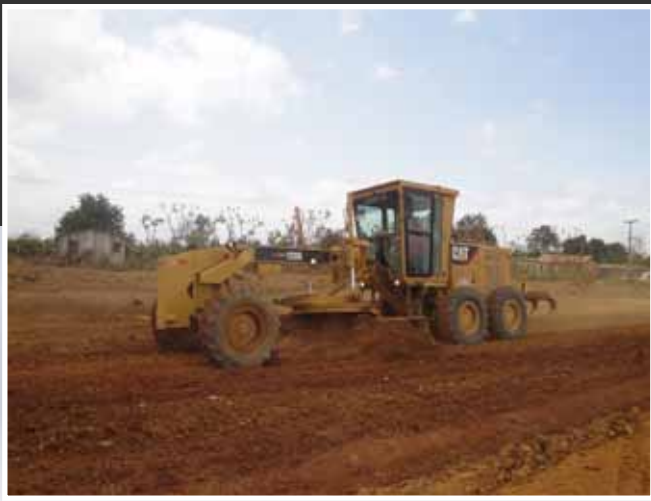
Mixing of EMC SQUARED System Stabilizer Solution with Subballast Soil Materials
