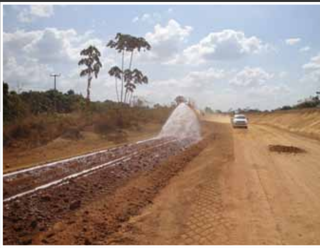
Application of EMC SQUARED® System Stabilizer Solution with Subballast Soil Materials
