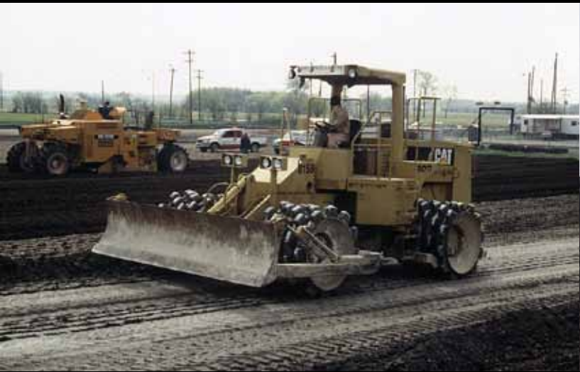
Compaction of Treated Clay Soil
