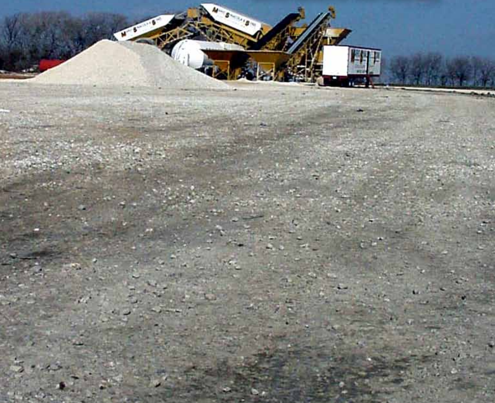
Stabilized Concrete Batch Plant Site One Year After Stabilization With Scattered Aggregate Remaining From Footprint of Large Aggregate Stockpile
