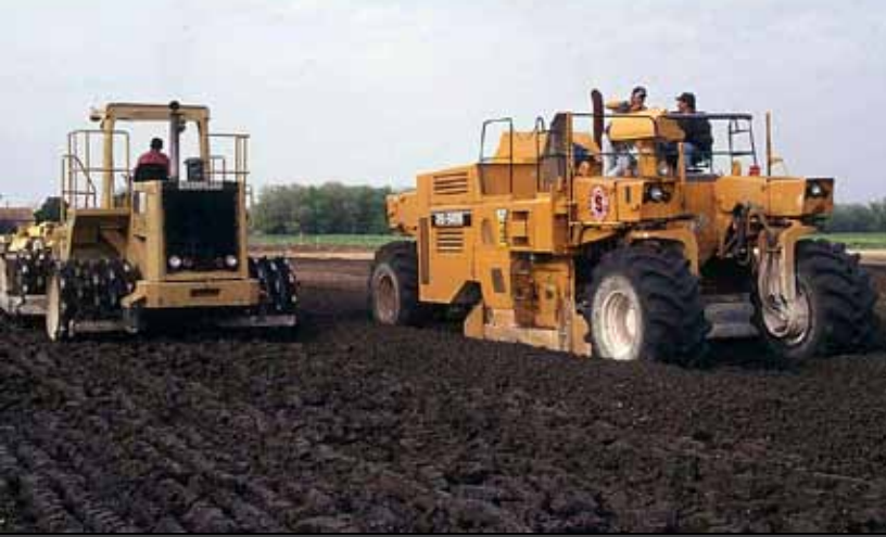
Mixing And Compaction of Treated Clay Soils
