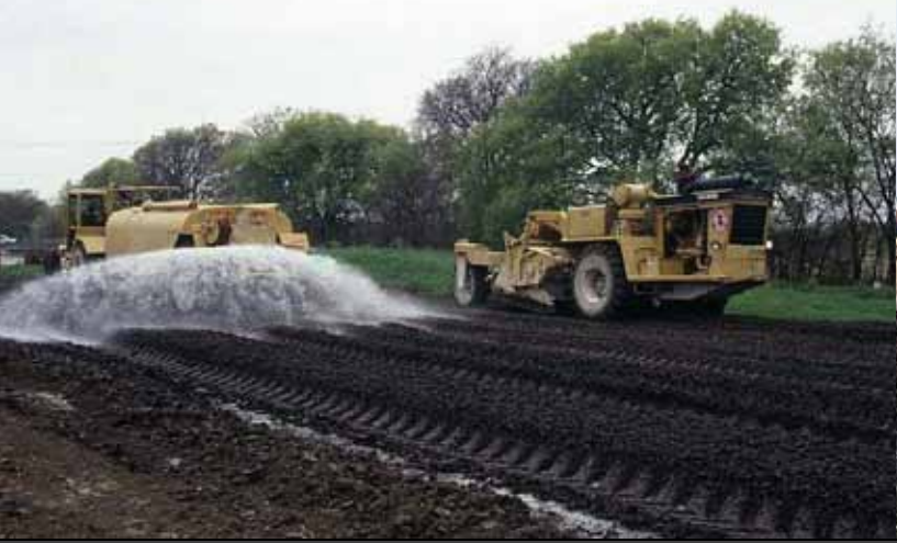
Application of EMC SQUARED® System Stabilizer Treatment
