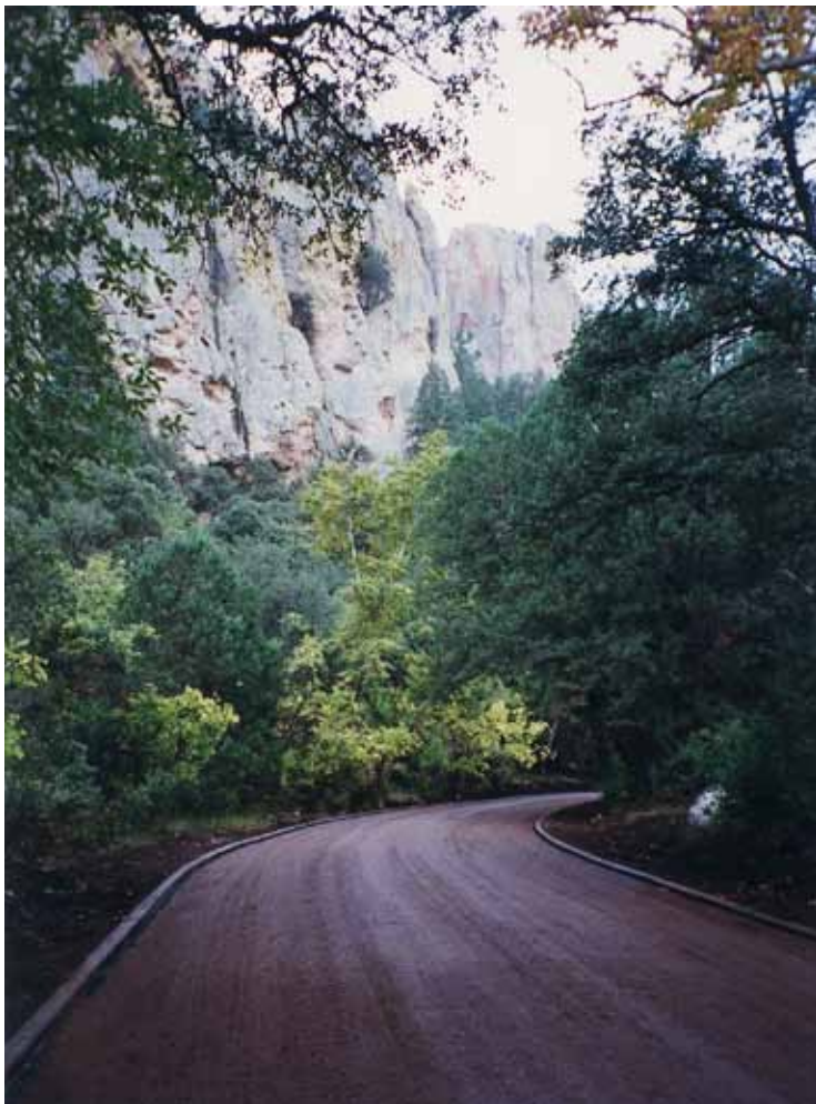
Road prepared for paving
